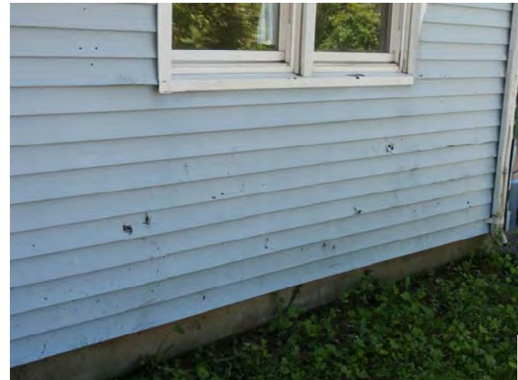
Example of common vinyl siding damage
