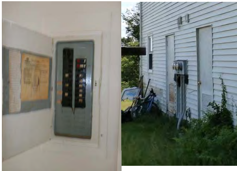
Typical circuit breaker panel and meter box
