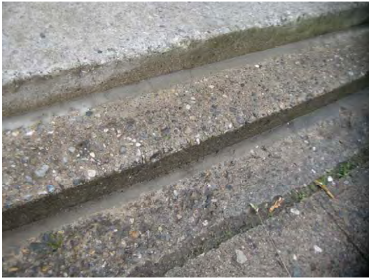
Typical example of concrete age related deterioration
